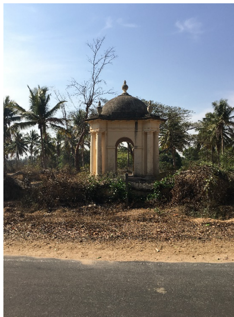
Proposed new gateway in the low curve of the perimeter wall, beside the concrete post.
